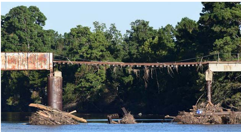
Union Pacific’s ex-SP “Rabbit” line bridge across the San Jacinto river near Humble was partially washed out due to flooding in the aftermath of Hurricane Harvey’s late August passage. The bridge has since been repaired and the line to east Texas has reopened. Photo by C. Randall Wilson
