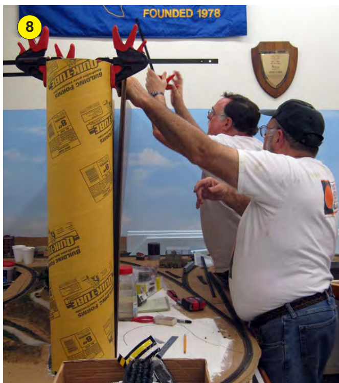
Photo 8: El Presidente Ted Davis and I are clamping masonite, having cut the board to size and opened the portals... measure once cut twice, no that's not it, it's the other way around! We tapered the end of the masonite to minimize the seam against the end tubes. We used 8-in. concrete form tubes to form the rounded ends.
