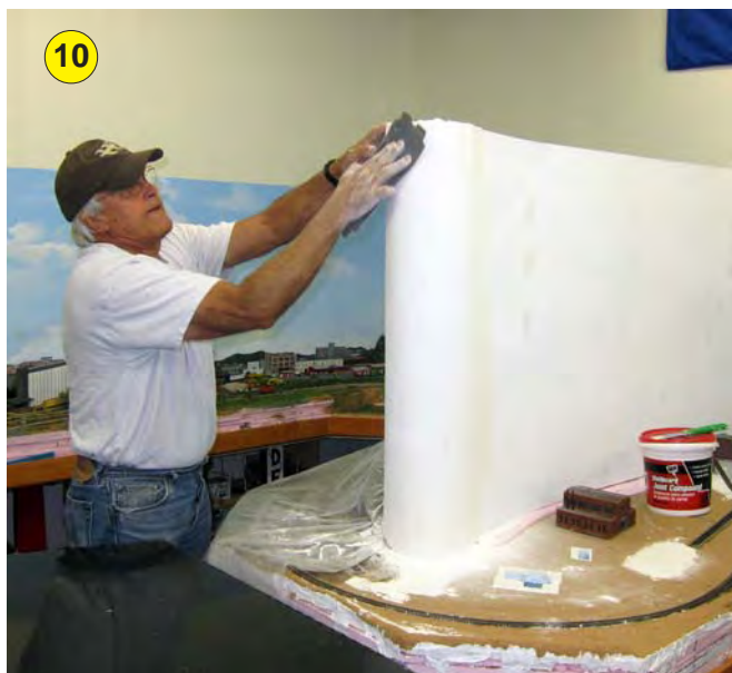
Photo 10: Glued, screwed, primed and now spackled with drywall mud: Terry Hooks sands the seams and makes sure to maintain the round appearance of the view block ends. After another coat of primer, he will paint the sky and clouds as he did all the way around the room.
